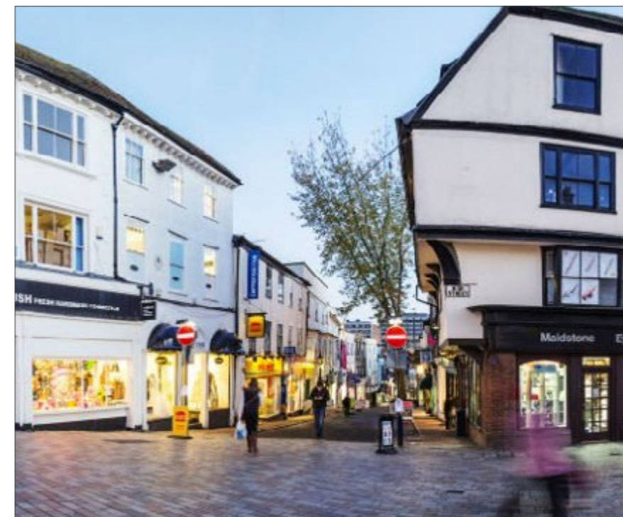
A mix of uses: Retail and residential uses mix well in town centres. Week Street in Maidstone town centre is a good example of this.
