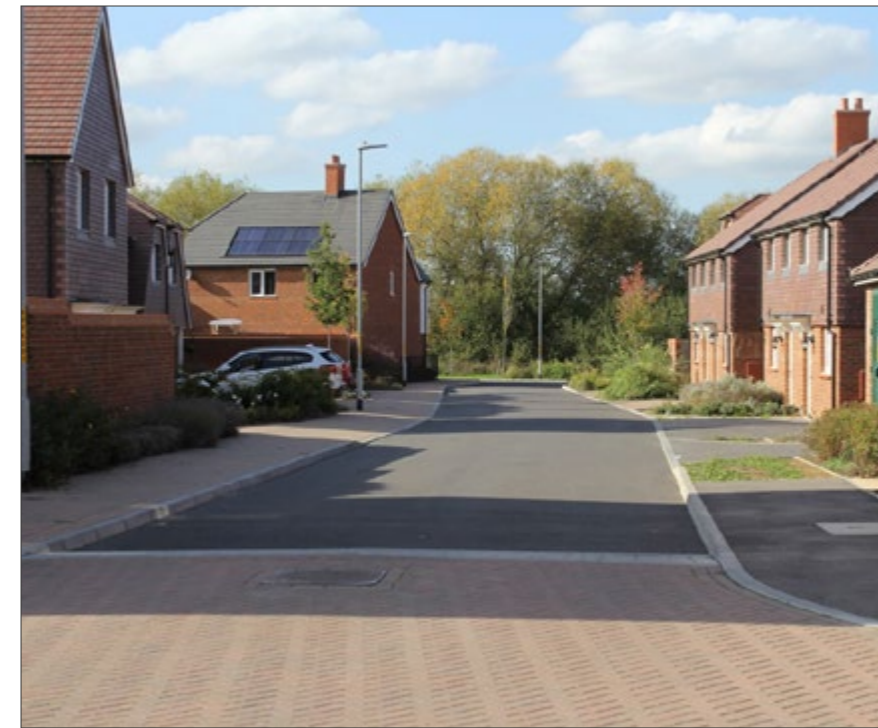
Visual connectivity: Make sure that people can see where routes lead to. Here, a strong visual connection between the main street at the front of the site and the park at the back helps people find the things they want.
