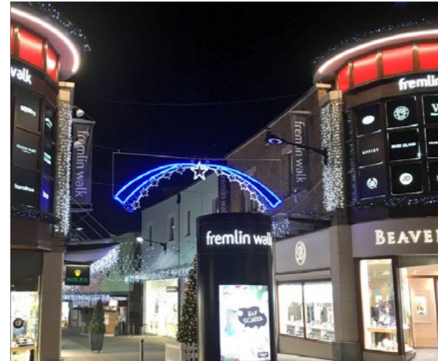
Active streets: Retail centres such as Fremlin walk maximise the activity along their edges, making the spaces between buildings vibrant and attractive.
