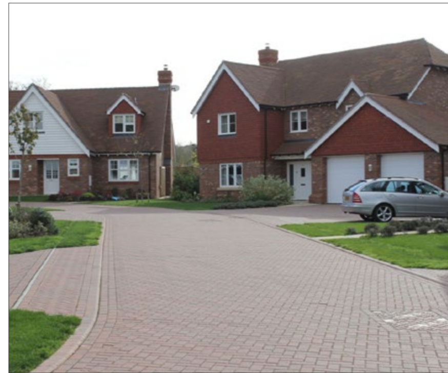
Shared surface: In places with very low vehicle movements (less than 100 per day) it may be appropriate to create a shared surface like this one.
