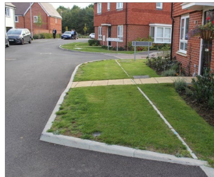
Accommodating services: Flat-laid blocks have been used to delineate the service strip at the edge of the carriageway. This creates the false impression of a footpath and should be avoided.
