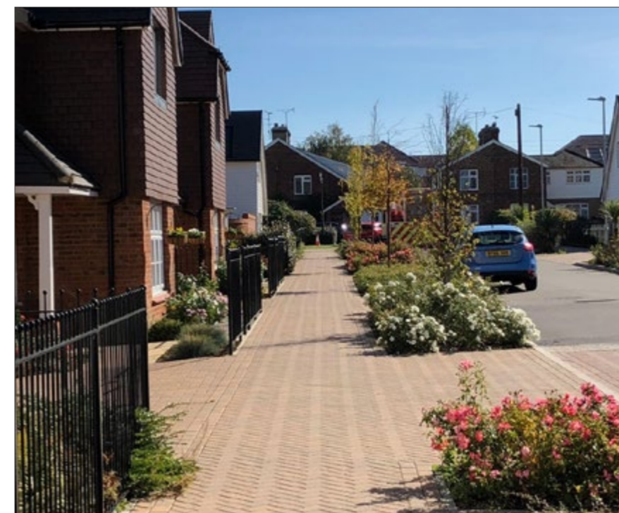
Managing water: The verges in the development double as part of the water management system. Plants absorb run-off, with excess water travelling along the swale to storage areas in the main square. This means that the technical requirement to manage surface water is performed in a way that provides an attractive amenity for residents. It also provides opportunities to improve biodiversity.
