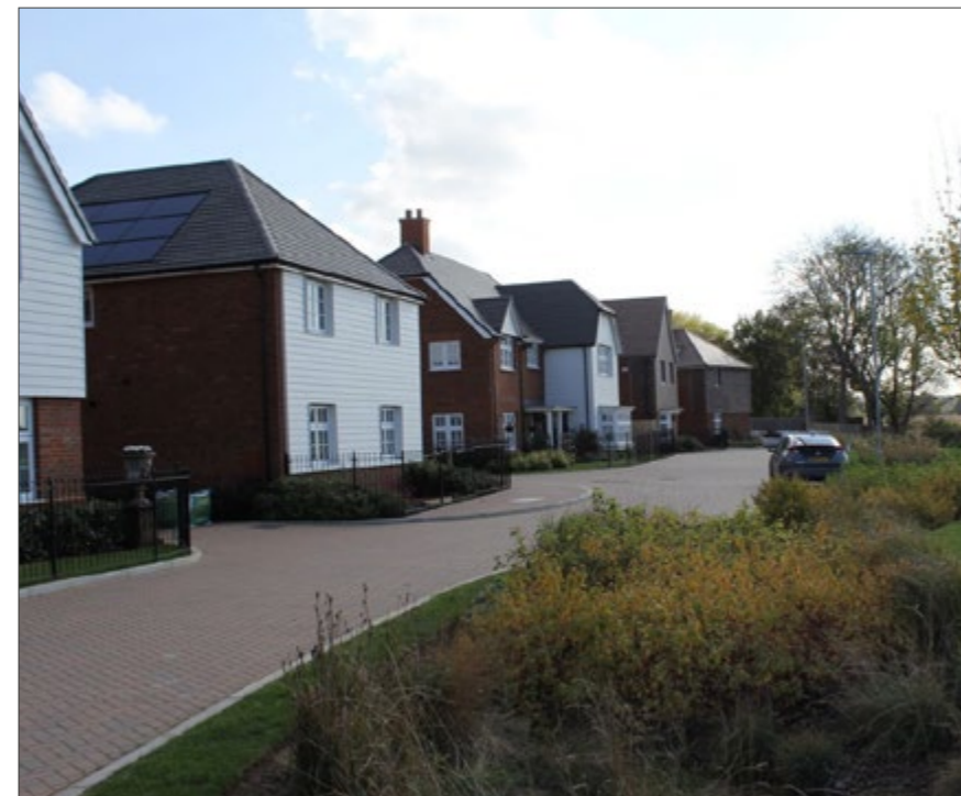
Keep an eye on drag distances: For private drives such as this one, bin collection points should be provided as often refuse collectors will not collect bins from properties along drives like this.
