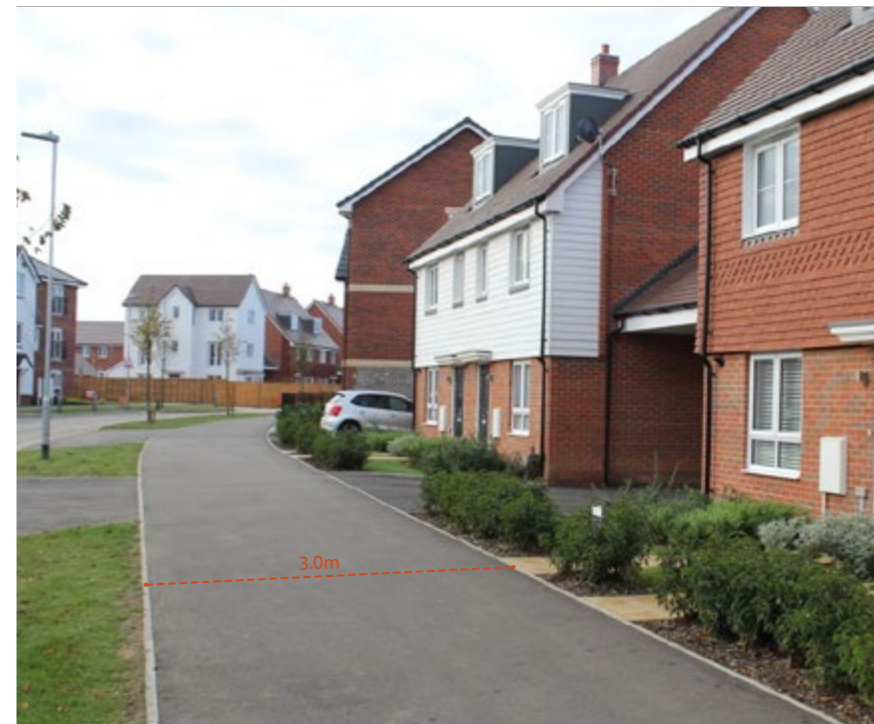
Shared footway / cycleway: Making surfaces wide enough so that both cyclists and pedestrians can be a good way to get less confident cyclists who are intimidated by main roads out on their bikes.
